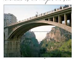
1863, during the reign of Napoleon III. This bridge is composed of four arches; the main arch is of 56 meters. "El Kantara" is 125 meters height above the Rhummel River and 128 m span...
