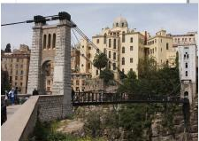
year 1907, on until the year 1912. It contains three main curves with 27 arches; the largest curve measures 70 meters. It is 447 meters span, 12 meters width, and 105 meters above the Rhummel River. "Sidi Rached" is classified among the highest bridges made of rocks in the world. Under the bridge "Sidi Rahed" is found "The Bridge of the Devil" ... It was given this name for the infer-
