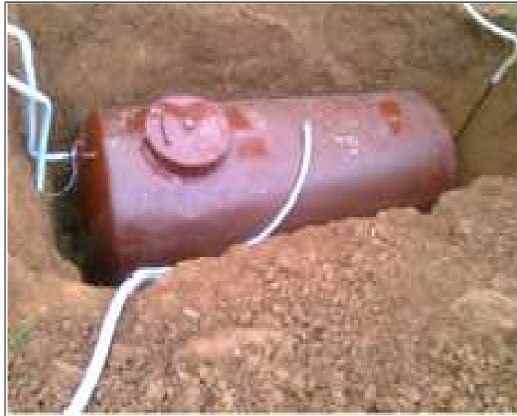
Fig.4: The tank embankment
